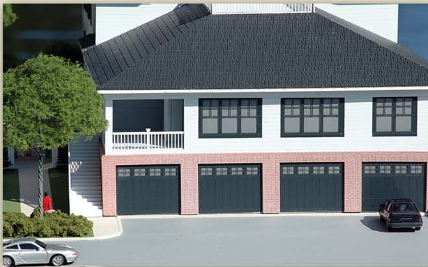
Meeting Park Condominium Residences Rear Elevation
